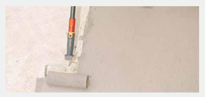
Technical features: ACQUASHIELD+ is a two-component mortar consisting of high resistance cements, fine aggregates with graded particle size (less than 0,3 mm), special additives (component A) and synthetic polymers in aqueous dispersion (component B).
